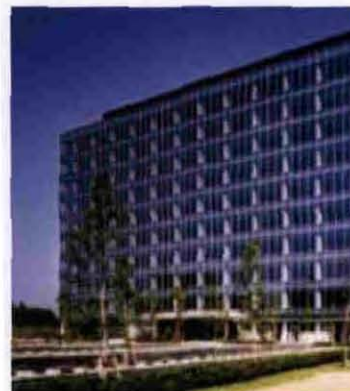
KDX Toyosu Grandsquare, Tokyo $367M
