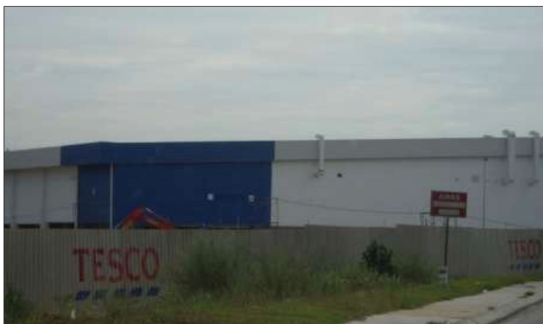
Figure 7: TESCO Shopping Complex (under construction)
