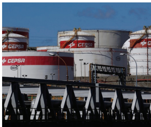
Carlyle: oil and gas facility: Spain
