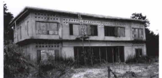
Figure 6: A detached house (under construction) in the Bangi, Malaysia endeavours to achieve Passive Architecture goals via wide openings facing north.
